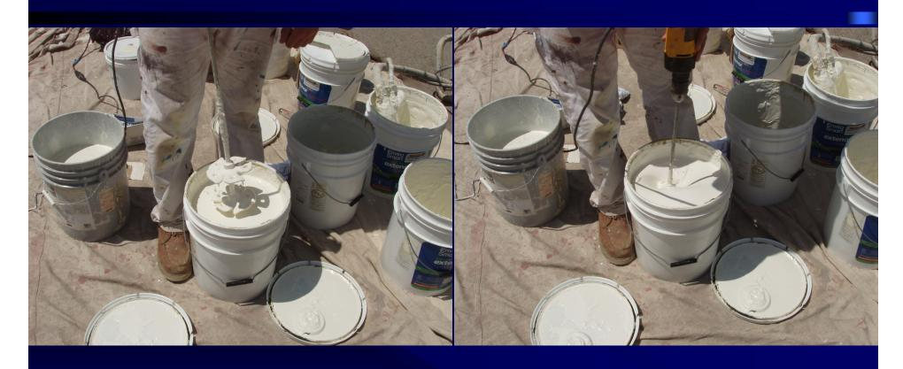
Drill Paint Mixer used to Stir Product On-Site
